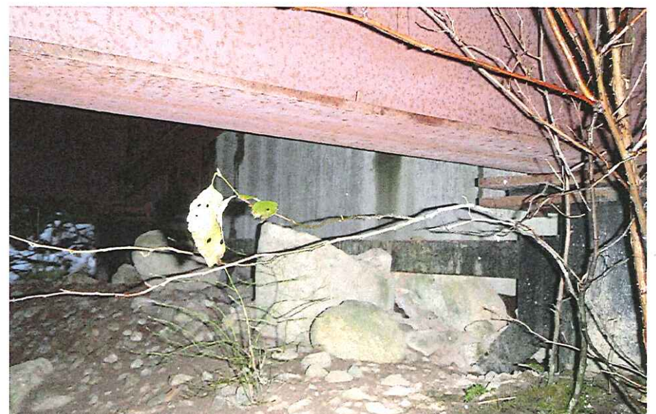
CK-2032 Abutment Right Bank
