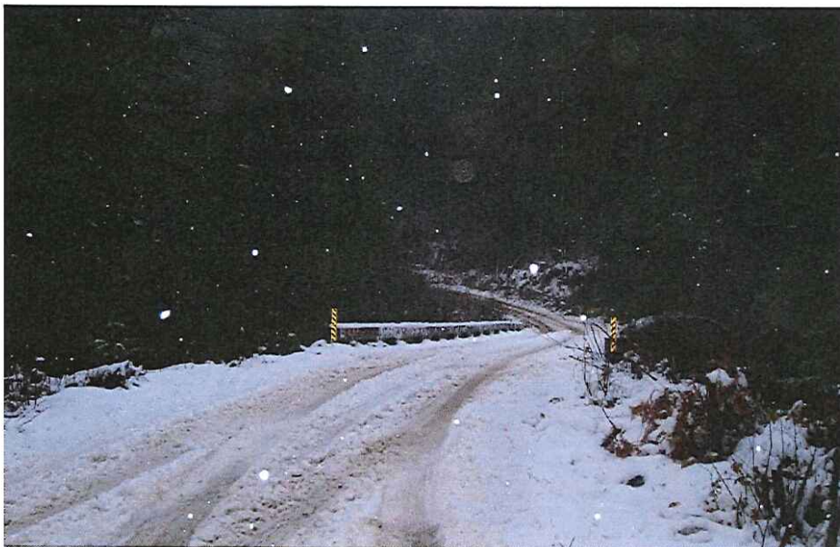
CK-2032 Approach Right Bank
