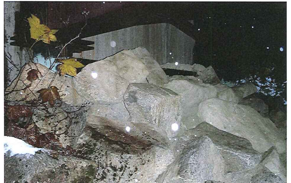
CK-2032 Abutment Left Bank
